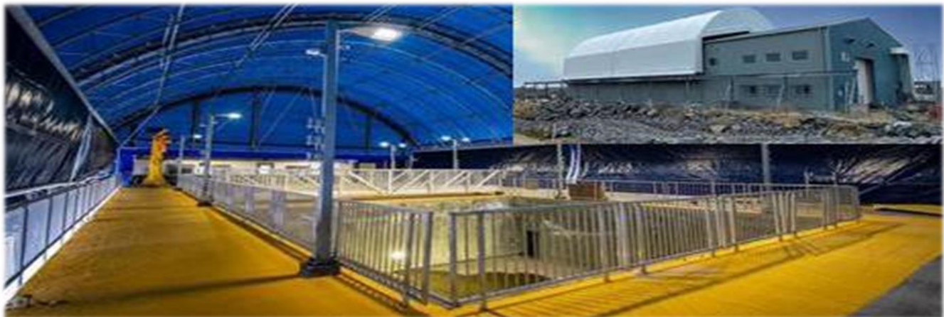
Figure 1. OSIM facility (inset, top-right) at CMO showing the seawater tanks and retractable roof for meteoric snow accumulation on natural grown sea ice from seawater piped in from Hudson Bay (background of inset image).
